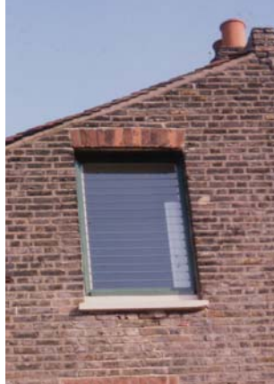
A) Window to kitchen
