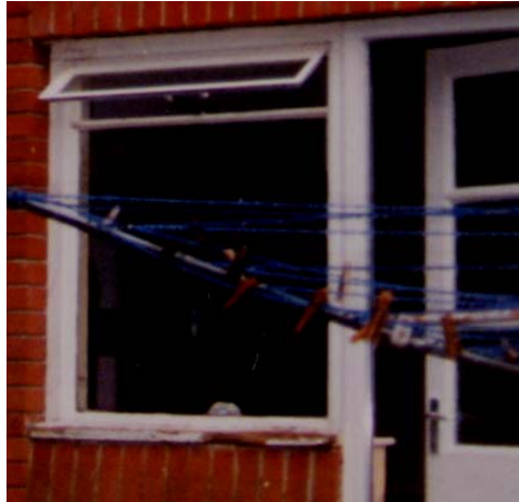
Ground floor rear kitchen/diner
