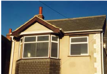
Closer view of main windows
