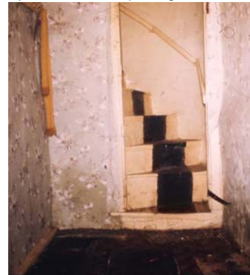
A) Stairs from GF passage
