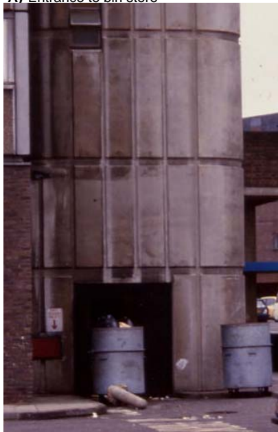
A) Entrance to bin store
